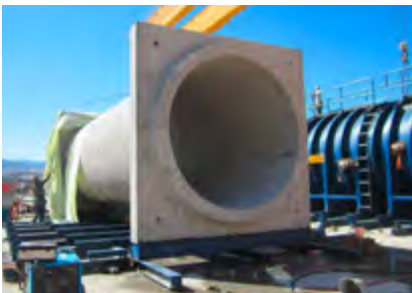
Shaft element pumped with UPP
