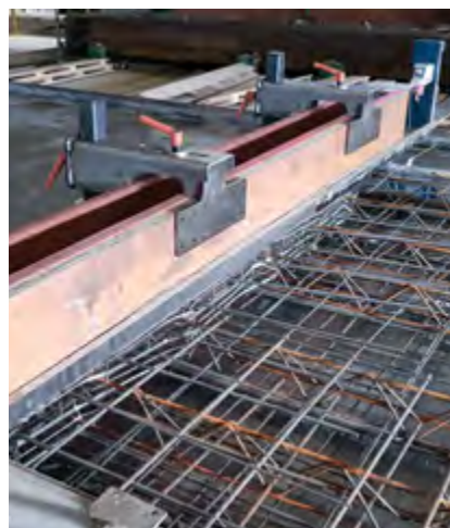
MST after concrete pouring
