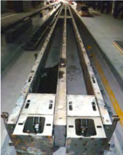
Pile shuttering based on the SAS-MF
