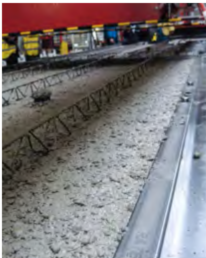
Girder slab production
