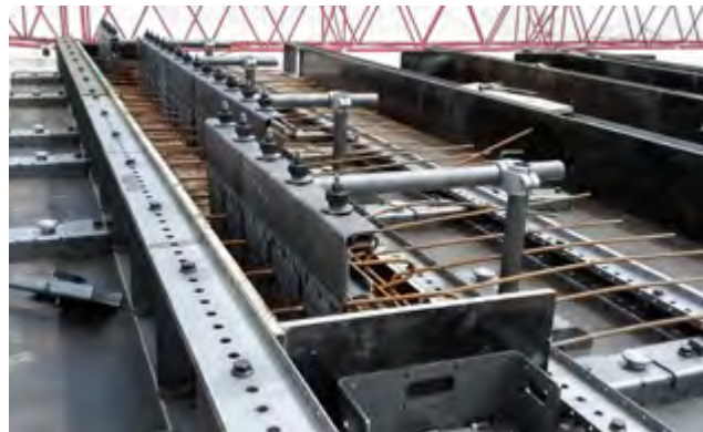
Easy Form in combination with UAR adapter
