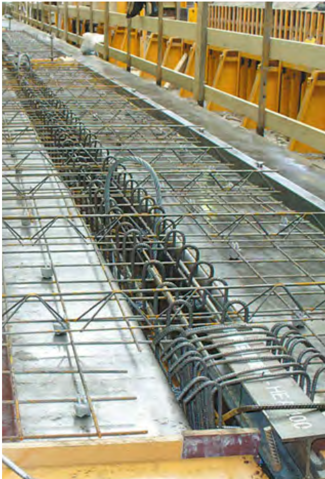
TT slab production
