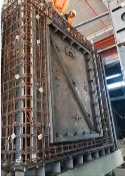
Shrinkable window shuttering
