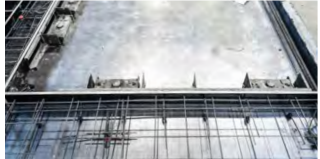
Recess with MST and wooden window corner
