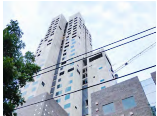
Facade elements, Indonesia
