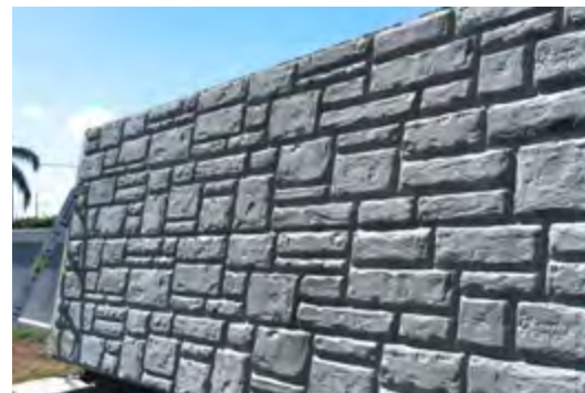
Noise barriers, USA
