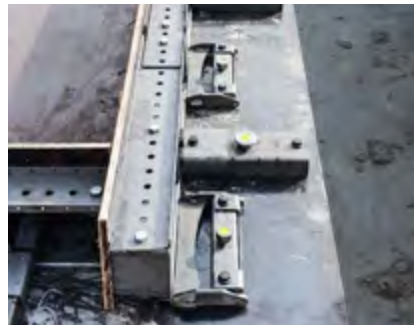
Easy Form with HT stop adapter
